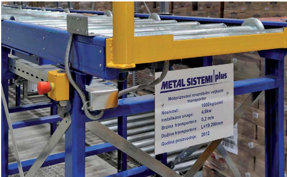
3-PL-Warehouse equipped with roller conveyors and METALSISTEM's "SUPER 4-5-6" Pallet Racking Series <October 2012>
