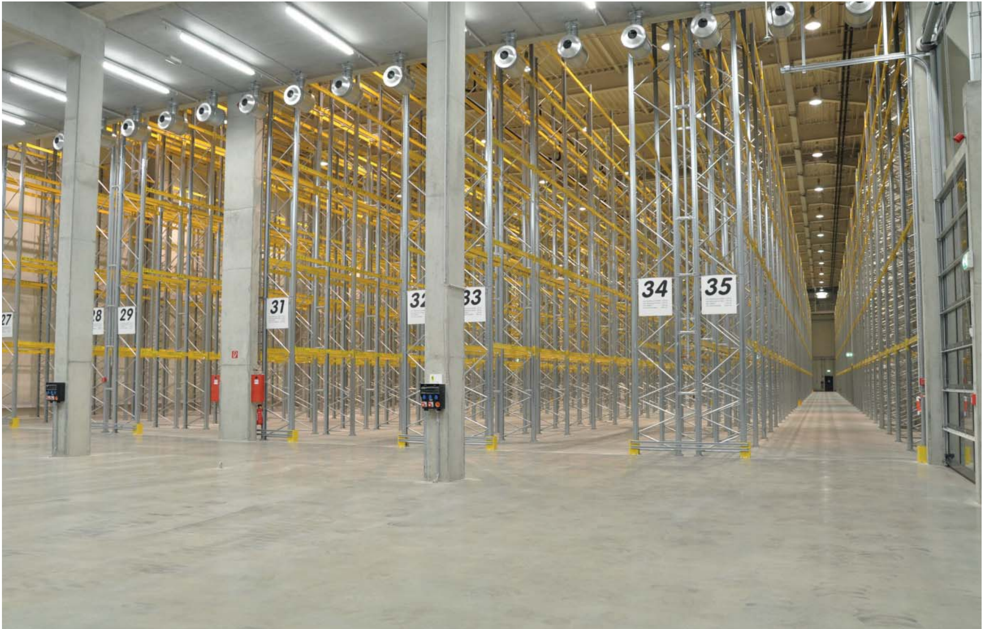
UNIBUILD Heavy Duty Pallet Racking Installation <July 2012>
