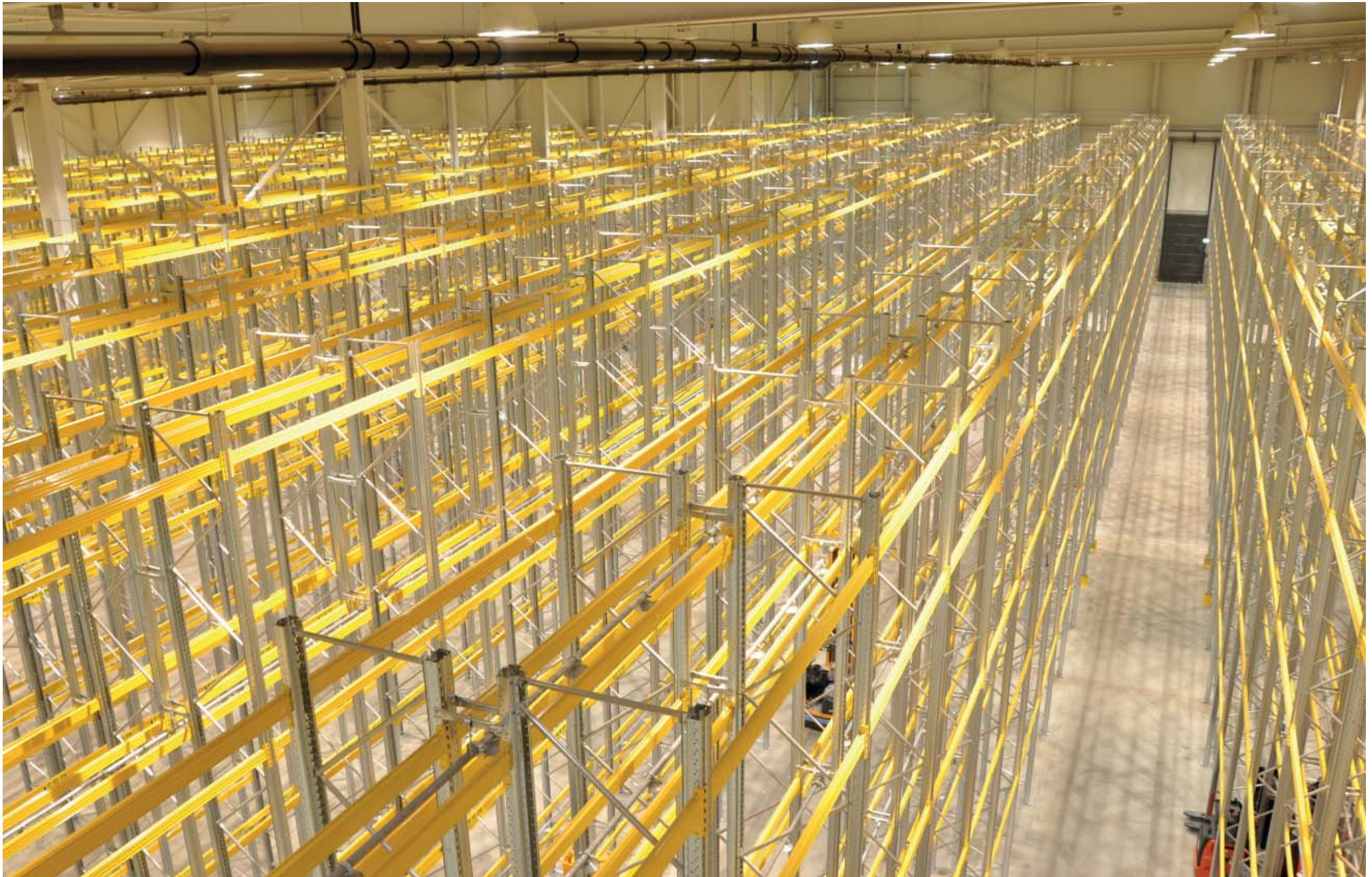
UNIBUILD Heavy Duty Pallet Racking Installation <July 2012>
