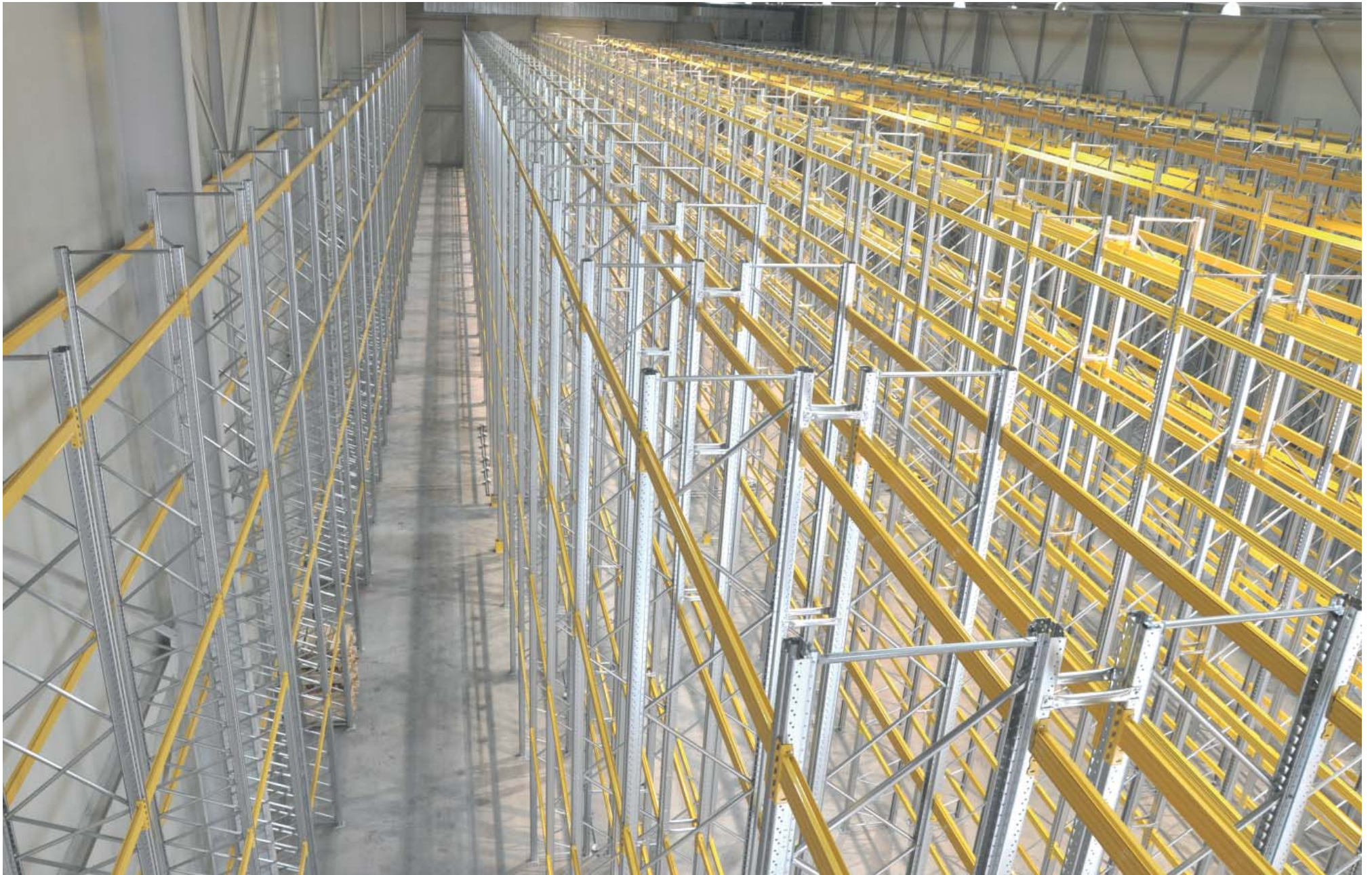
UNIBUILD Heavy Duty Pallet Racking Installation
