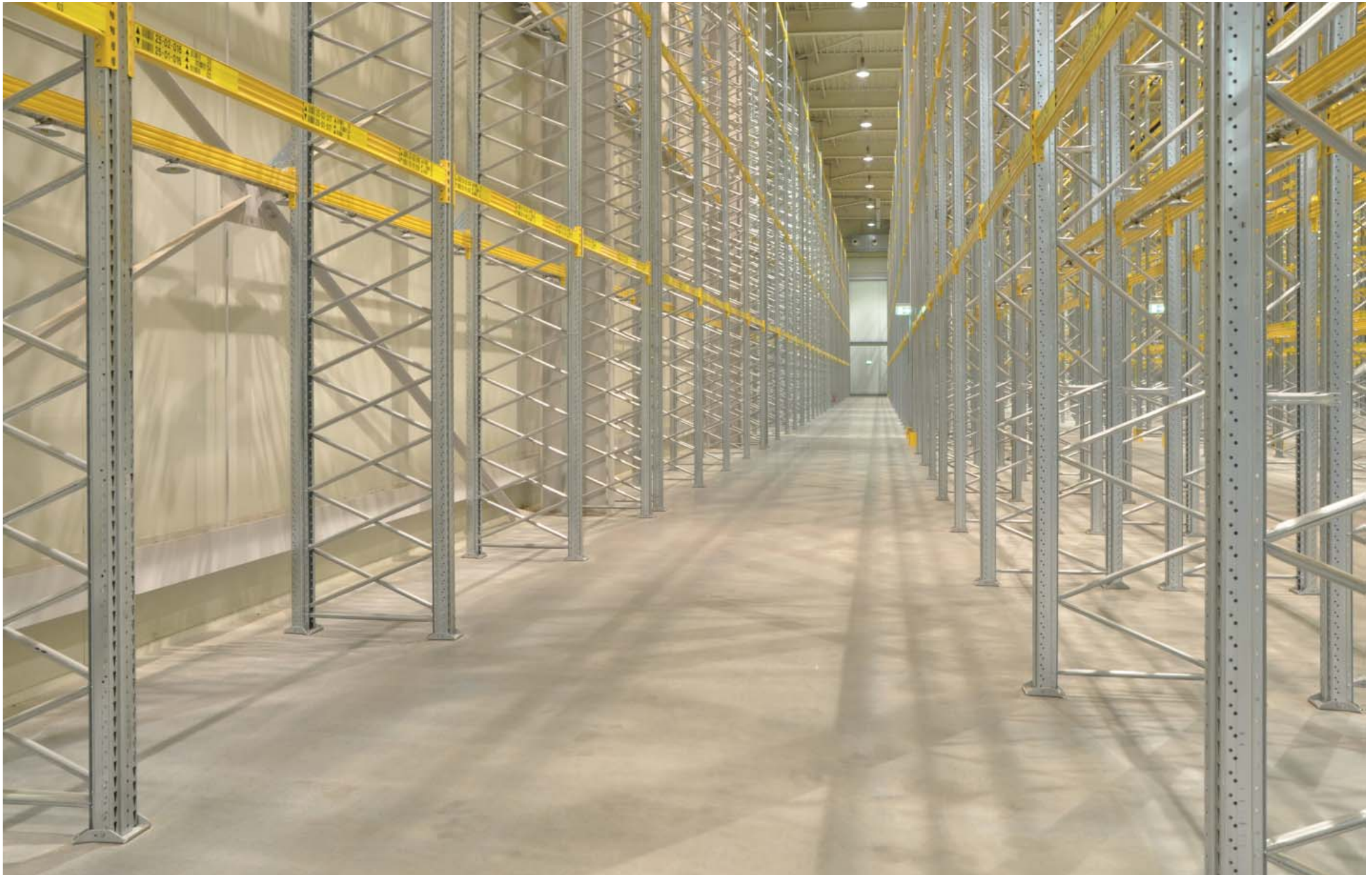
UNIBUILD Heavy Duty Pallet Racking Installation <July 2012>
